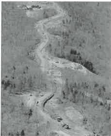
Figure 1.7: Road construction on Lowell Mountain in Vermont. Construction roads for vehicles must be 40 feet wide and highly compacted, creating contamination and runoff problems for local wildlife.
